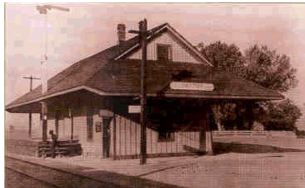
Dayton's Carson & Colorado Railroad Depot, approximately 1910, which would make it at that time the Southern Pacific Depot.
